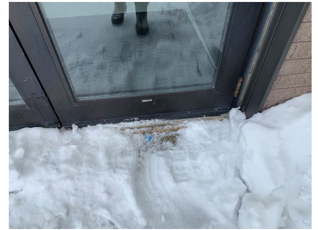
Door #14 Concrete Stoop
