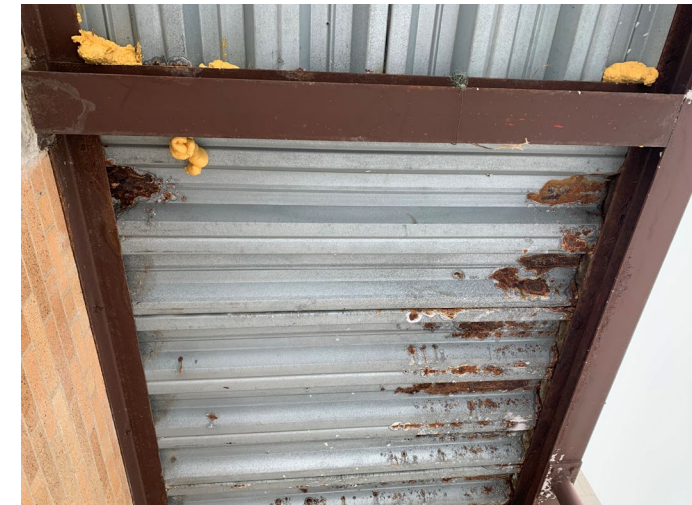
Door 7 and 8 Canopy
