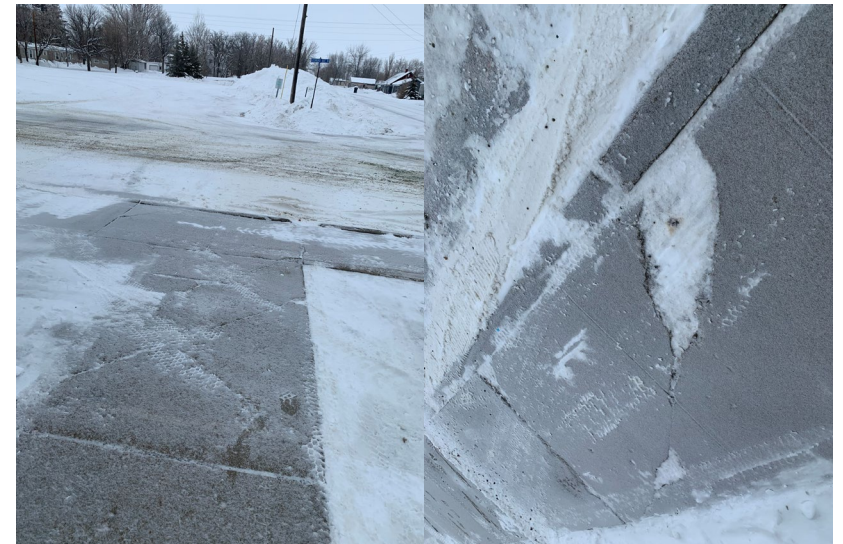
East Side Sidewalk Replacement
