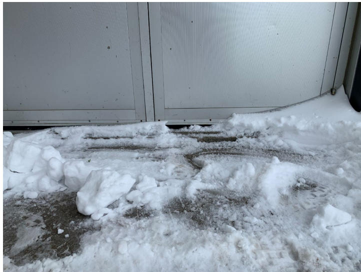
Door #15 Concrete Stoop
