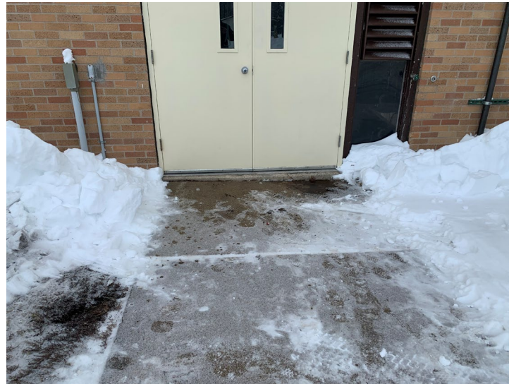
Door #16 Concrete Stoop
