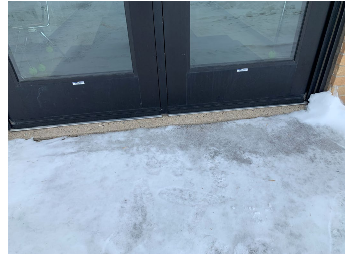
Door #4 Concrete Stoop
